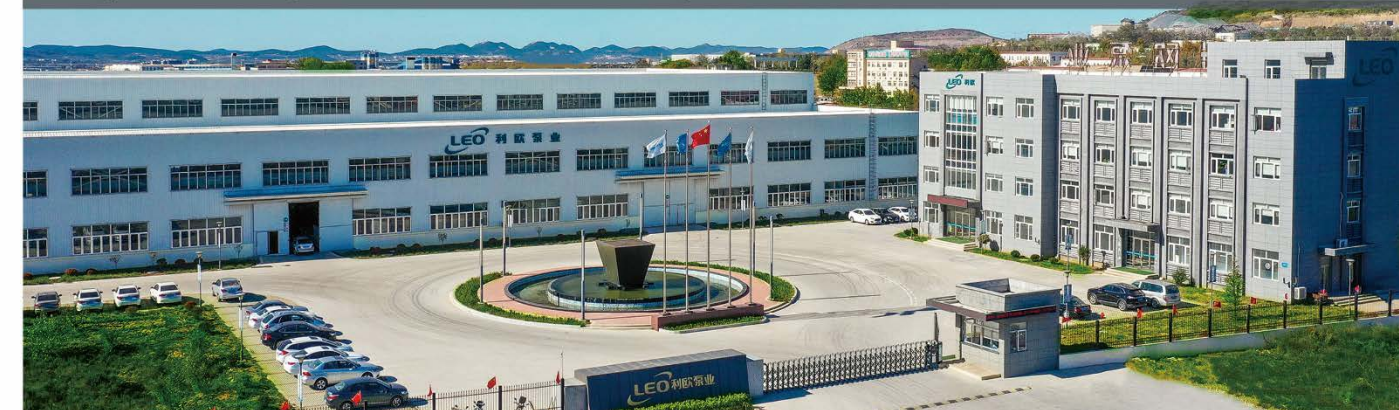
Pump Manufacturing Base for Petrochemical Industry
